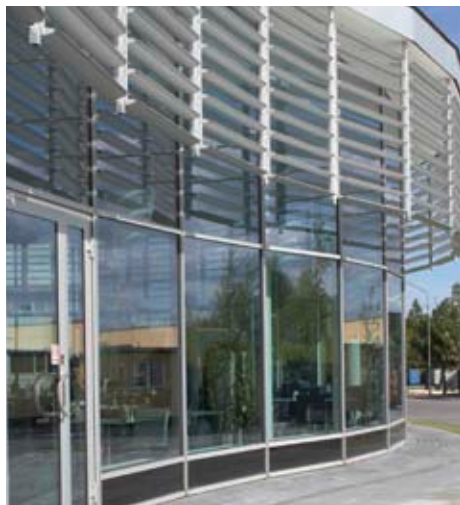
Effective solar shading maintains translucency and brightness in rooms without them heating up too much.
