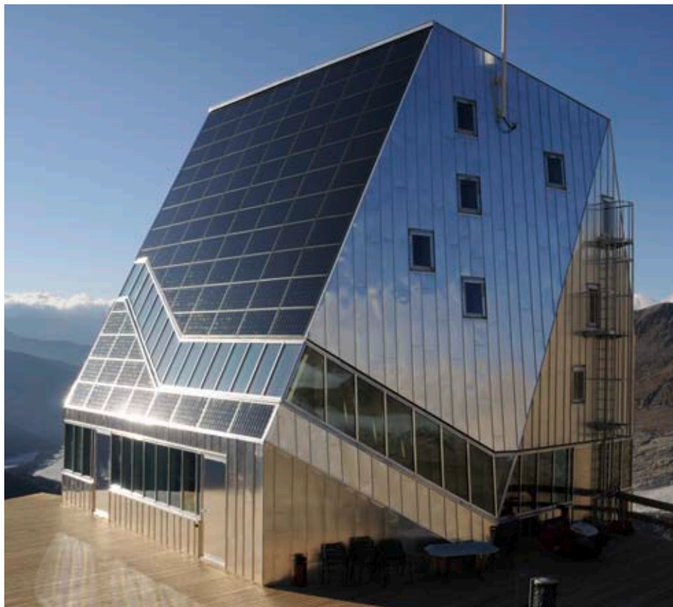
Aluminium offers more than just a roof over one’s head, even under extreme conditions; the Monte Rosa mountain hut, which has won an award for self-sufficiency, is shown here.
